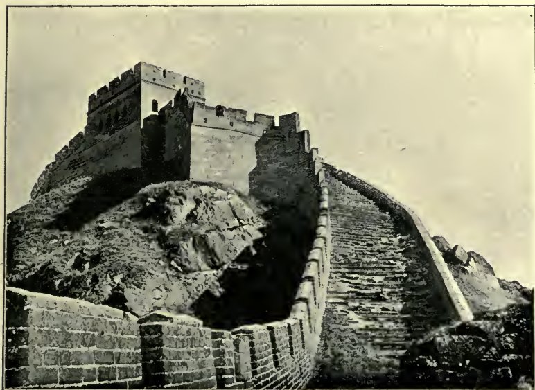
A WATCH-TOWER ON THE GREAT WALL
